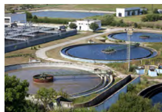
Municipal Water Treatment
